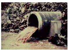
Illicit discharge example - Sediment laden runoff
